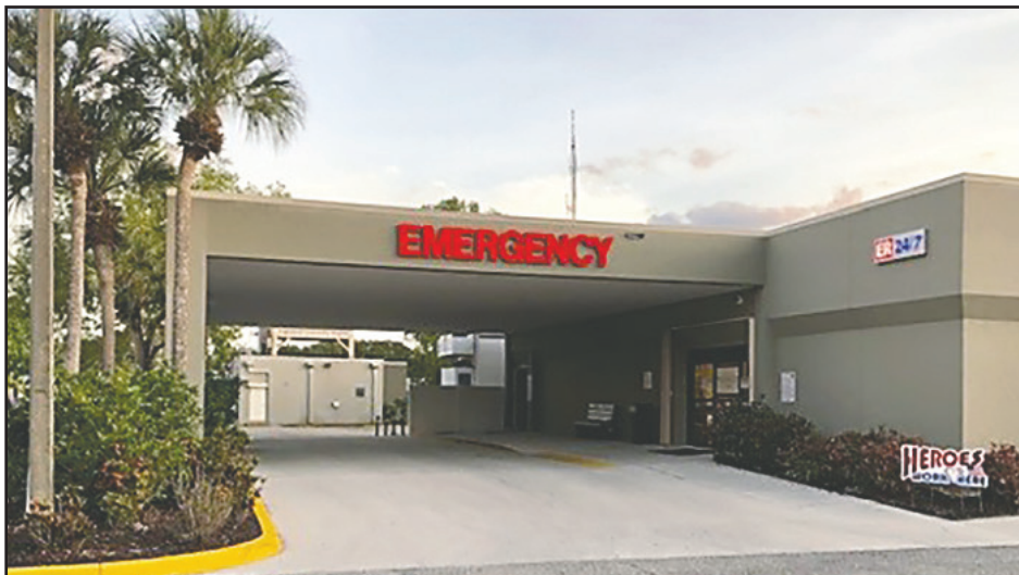
Englewood Hospital's emergency entrance at the rear of the main building is well marked.
