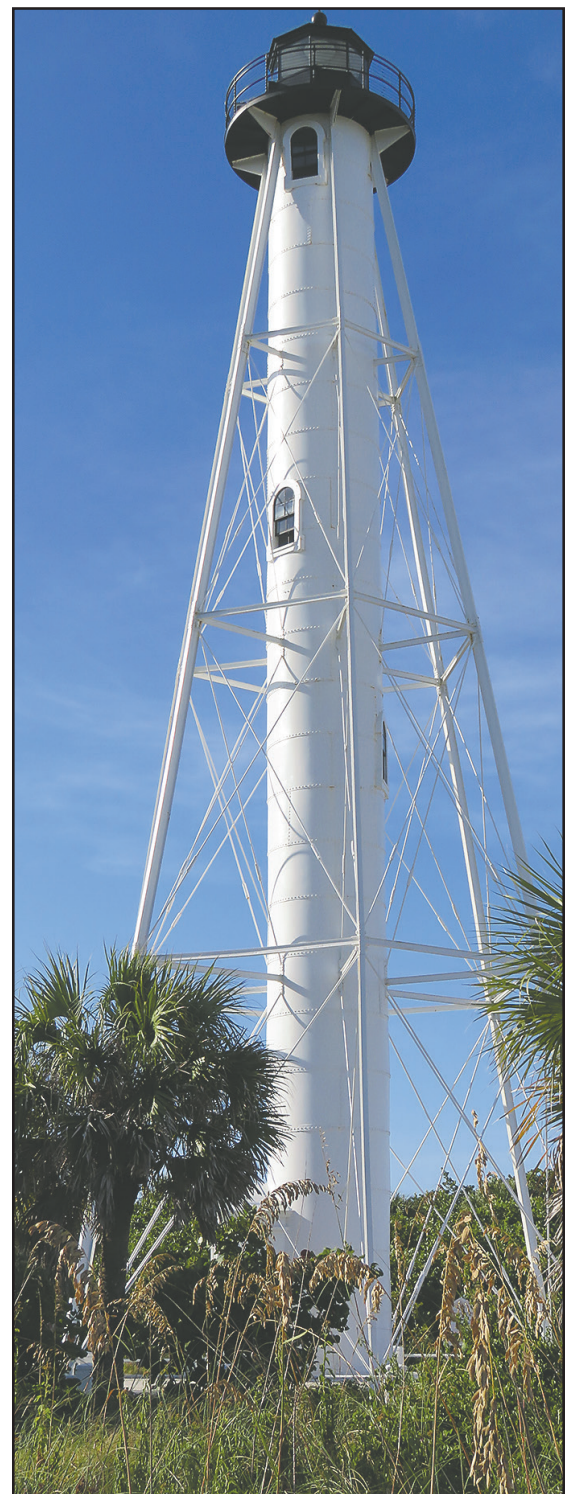
The restoration of the Gasparilla Lighthouse was accomplished thanks to BIPS.
