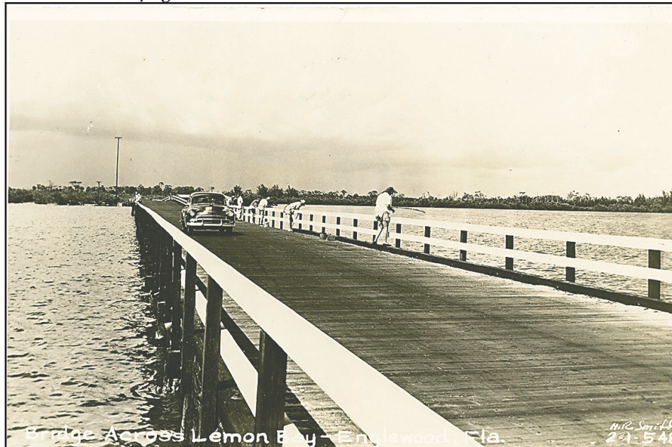
The Chadwick Bridge across Lemon Bay.
