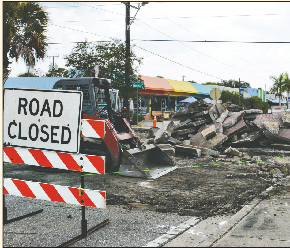
Construction has started on West Dearborn Street.
