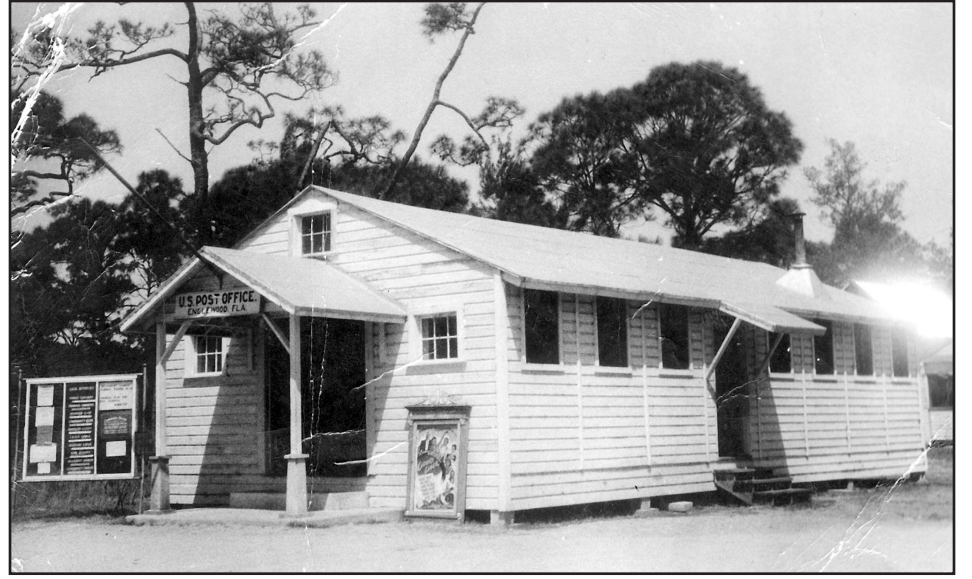
The Englewood Post Office, which was originally an army barracks at the Venice Airbase, was located at the northwest corner of Elm and Dearborn Streets.
