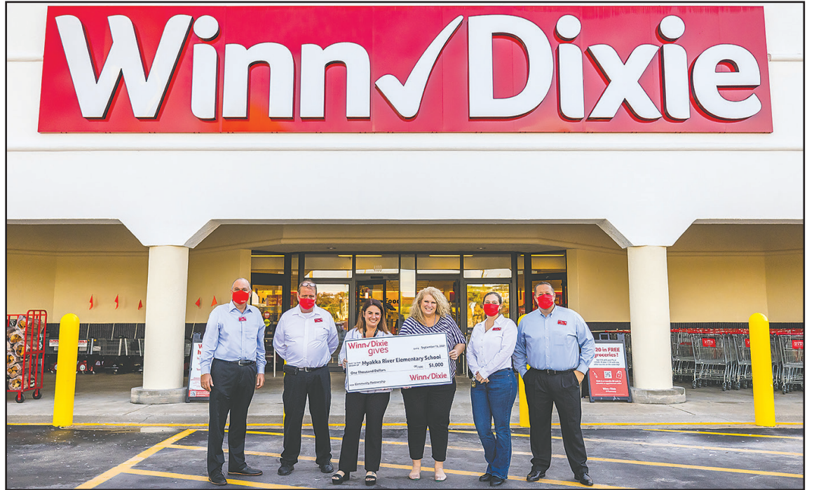
Winn-Dixie officially unveiled the newly remodeled Sunnybrook Winn-Dixie store and liquor store to the Englewood community with a ribbon cutting ceremony on September 15th. In celebration of the new store and to give back to the local youth and future leaders of the community, Winn-Dixie presented a $1,000 donation to Myakka River Elementary School during the ceremony. Over the past year, Winn-Dixie (WD) gathered feedback directly from local customers and associates to transform the Sunnybrook store into a convenient shopping destination that is both functional and beautiful for the local Englewood community. The refreshed Sunnybrook store now offers an updated produce department, an expanded deli and bakery, a new Dollar Shop within the store and much more for customers - all at the right price. To explore Winn Dixie online, go to www.winndixie.com . Pictured here (left to right): WD Regional Vice President Jorge Cabo, WD Store Manager Craig Clemons, Myakka River Elementary School Principal Grace Shepard; Myakka River Elementary School Lead Teacher Carrie Dillmore, WD Customer Service Manager Bridget Warner, and WD District Manager Kevin Lane.
